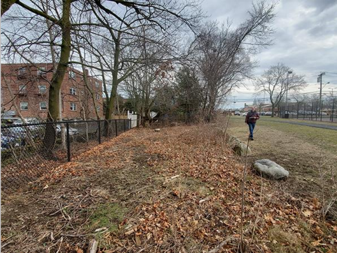
Flood Storage Area 2
