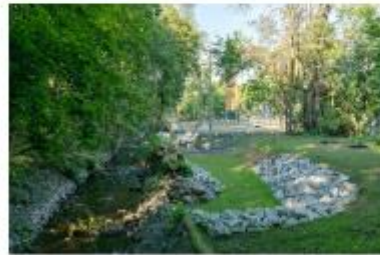
Photographs of the new boardwalk and natural flood storage area built in the first phase of construction. Credit: David Nussina.
