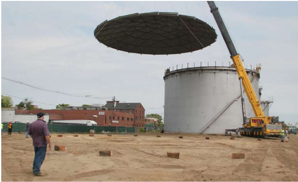
REMOVING THE TANK'S DOME ROOF
