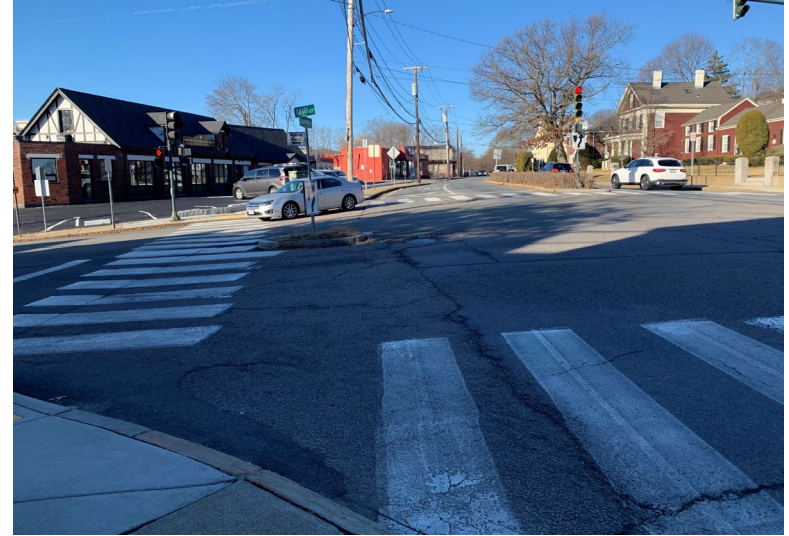
Mill St intersection has medians, turn lanes, wide receiving lanes
