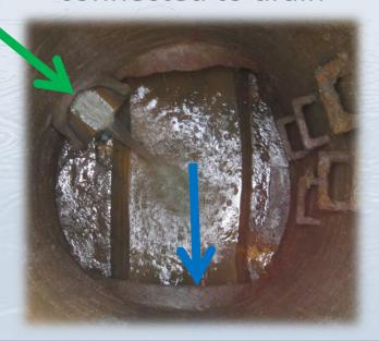
Top of municipal sewer broken to allow overflow to drain
