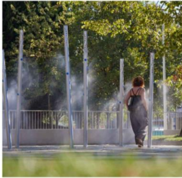
HEAT MITIGATING MISTING STATIONS
